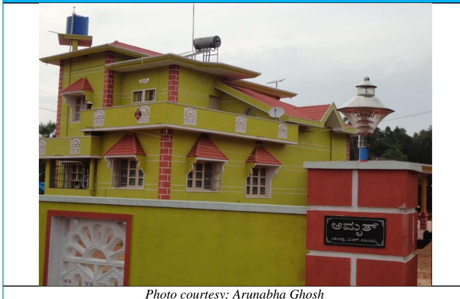
Photo 1.1: Installed SHW system in a rural home in Udupi district, Karnataka
